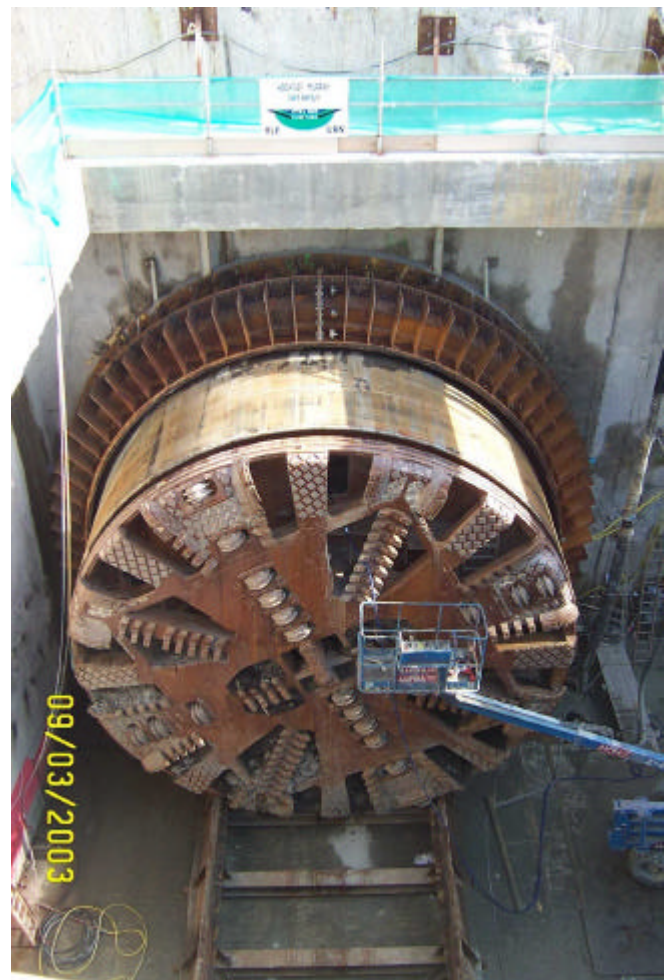
TBM after arriving at Thurrock portal
