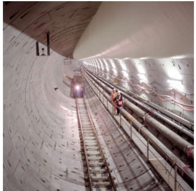
First Thames crossing tunnel
