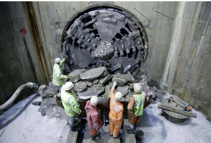
Dartford Lovat Machine at Reception Shaft by courtesy of National Grid
