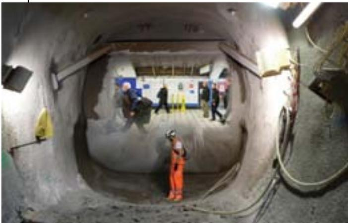
completion of the remainder of the jamb frame. All steelwork was installed using air winches and snatch blocks with appropriate holding down bolts which were secured onto the shotcrete.
