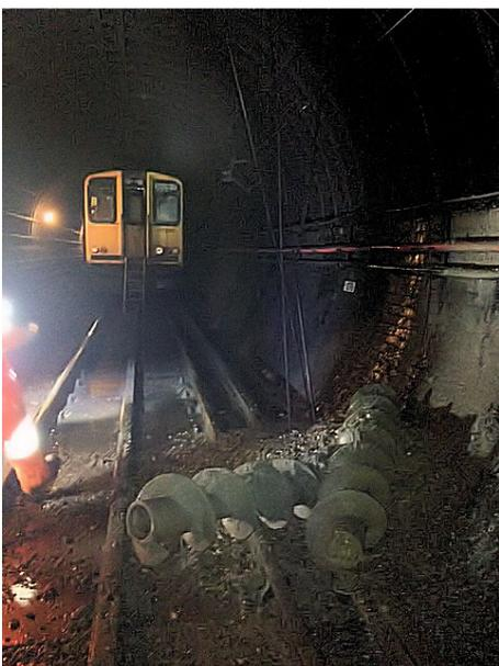
Figure 1: CFA auger sections found on the track after penetrating tunnel.
